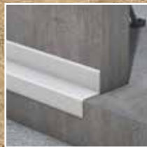
Connection joint between of precast elements
